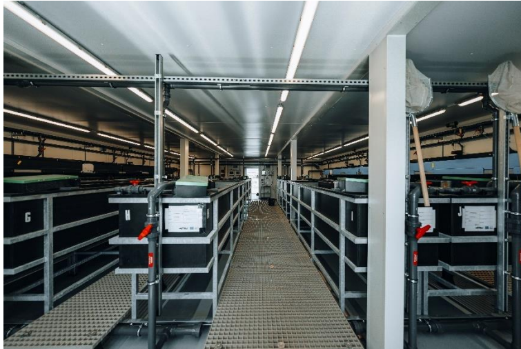
Figure 2: Hatchery container on the LIFE-Boat for rearing juveniles. © Julia Altpfart
